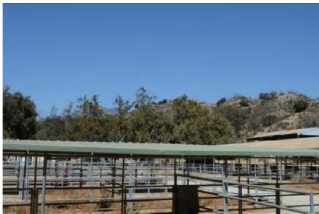
Demolish stables and cap all water supply pipes
