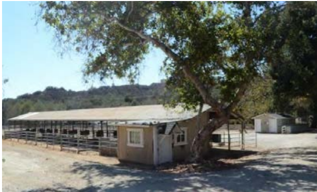
Demolish office and caretaker buildings, storage rooms, cap or remove septic tank(s)
