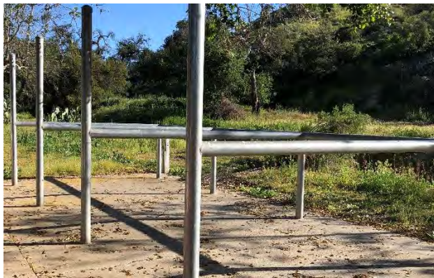
Demolish horse wash-out areas and other miscellaneous improvements onsite
